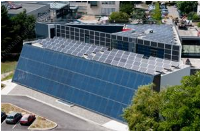
Fig. 1. Aerial view of the ADREAM building
