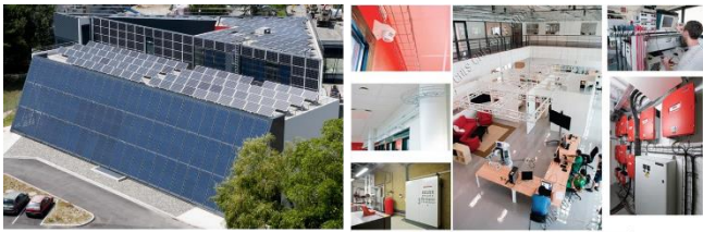
Figure 2. ADREAM BiPV installations, experimental rooms and sensors and monitoring systems
