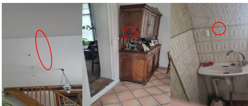
Figure 4. Example of sensors installation in the house
