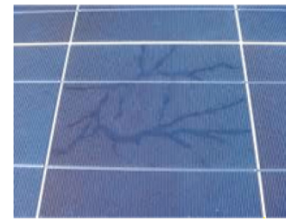
Fig. 1. Example of snail trail fault. Note the visual similarity with the trail of a snail.
