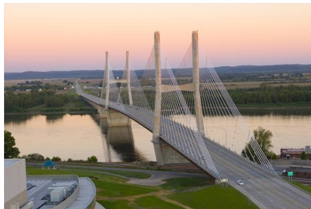
Figure I. 3: Pont Bill Emerson Memorial, Missouri – USA
