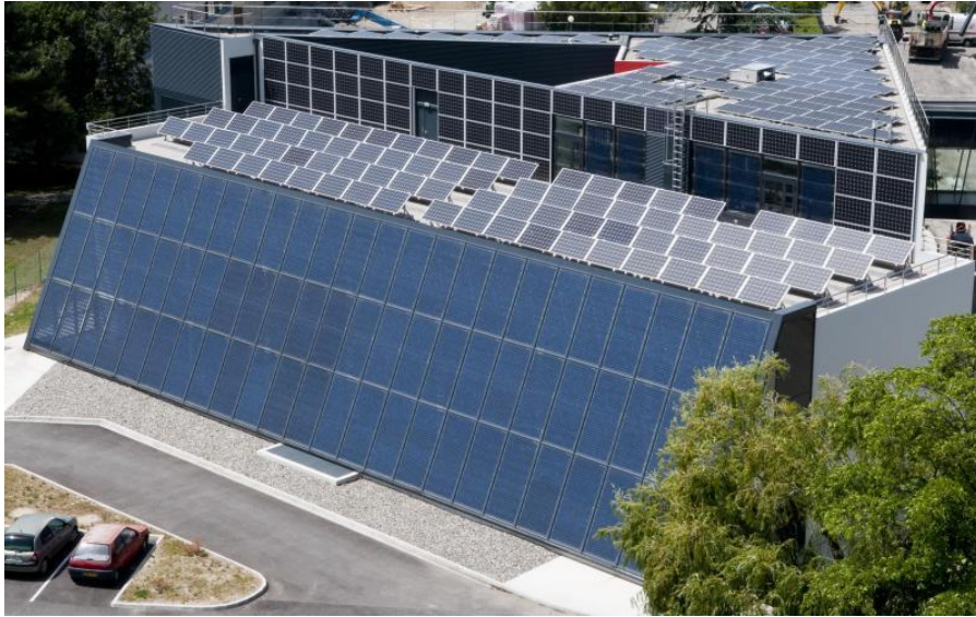
Figure 2.25 ADREAM building of the LAAS-CNRS
