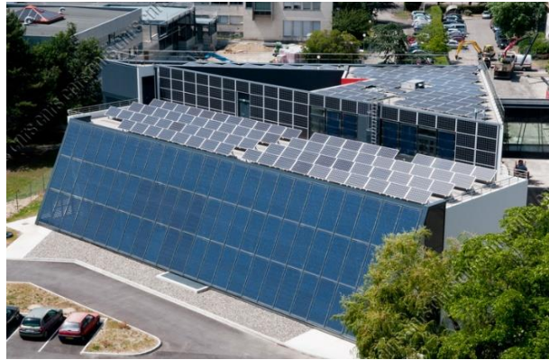
Figure 13: Aerial view of the ADREAM building in LAAS-CNRS
