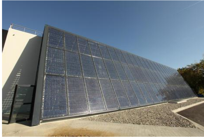
Figure 15: Double and triple glazing PV façade of the ADREAM building
