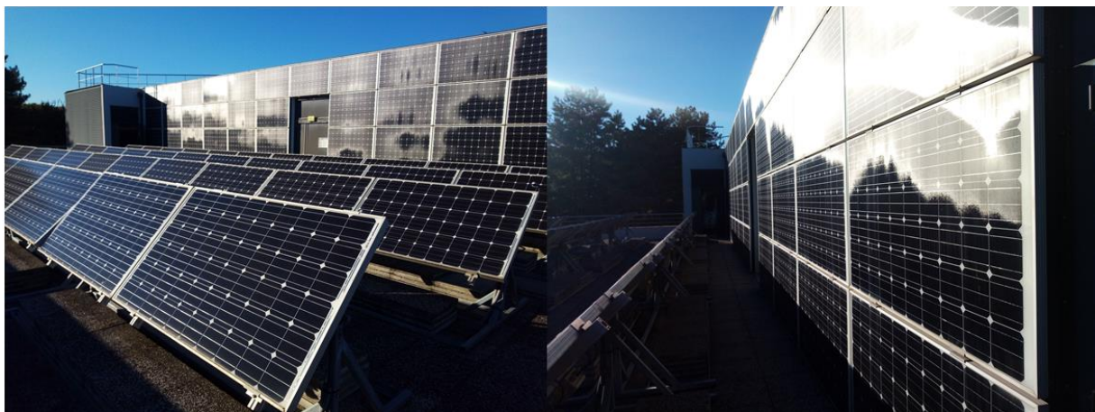
Figure 14: Regular crystalline silicon PV cells installed on the terrace and walls of the ADREAM building
