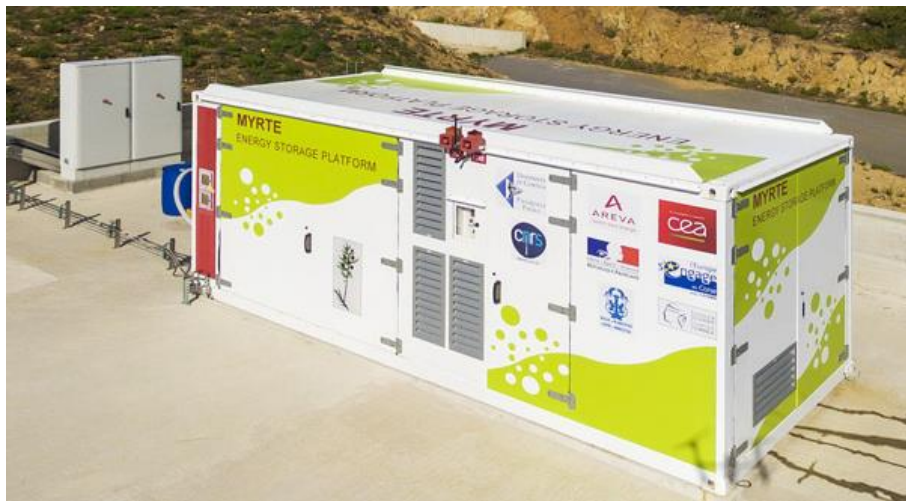
Figure 69: Electrolyser station for solar Hydrogen production of the MYRTE platform in Ajaccio
