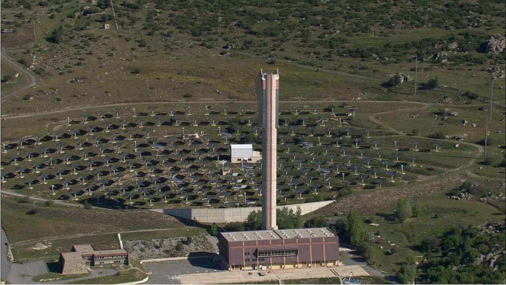
Figure 7: THEMIS concentrated solar plant [12]
