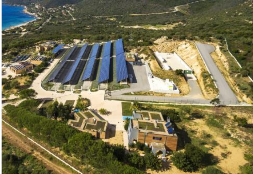
Figure 68: Solar PV installation of the MYRTE platform in Ajaccio
