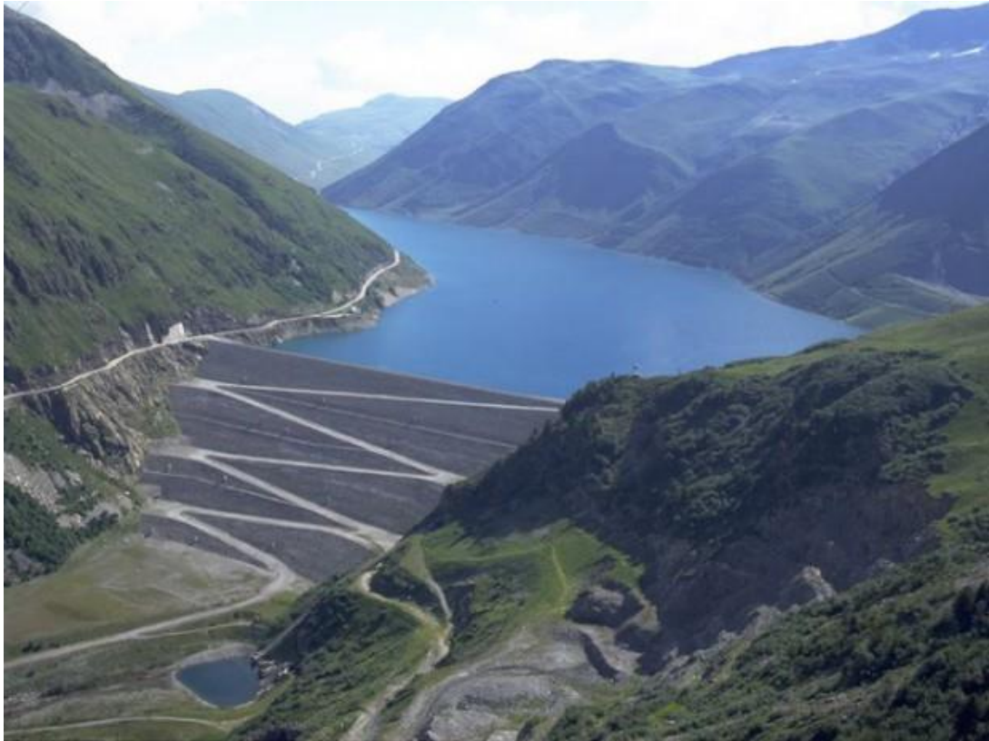
Figure 10: Picture of Grand'Maison Dam, the biggest pumped storage installation in France []
