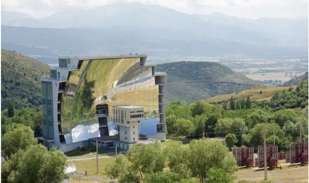
Figure 8: Concentrated solar Furnace ODEILLO, France [13]
