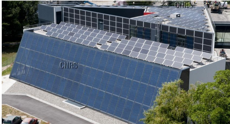
Figure 3.5: Aerial photography of the ADREAM building
