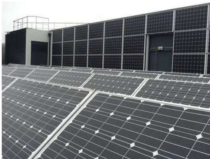
Figure C.1 Terrace of the ADREAM building
