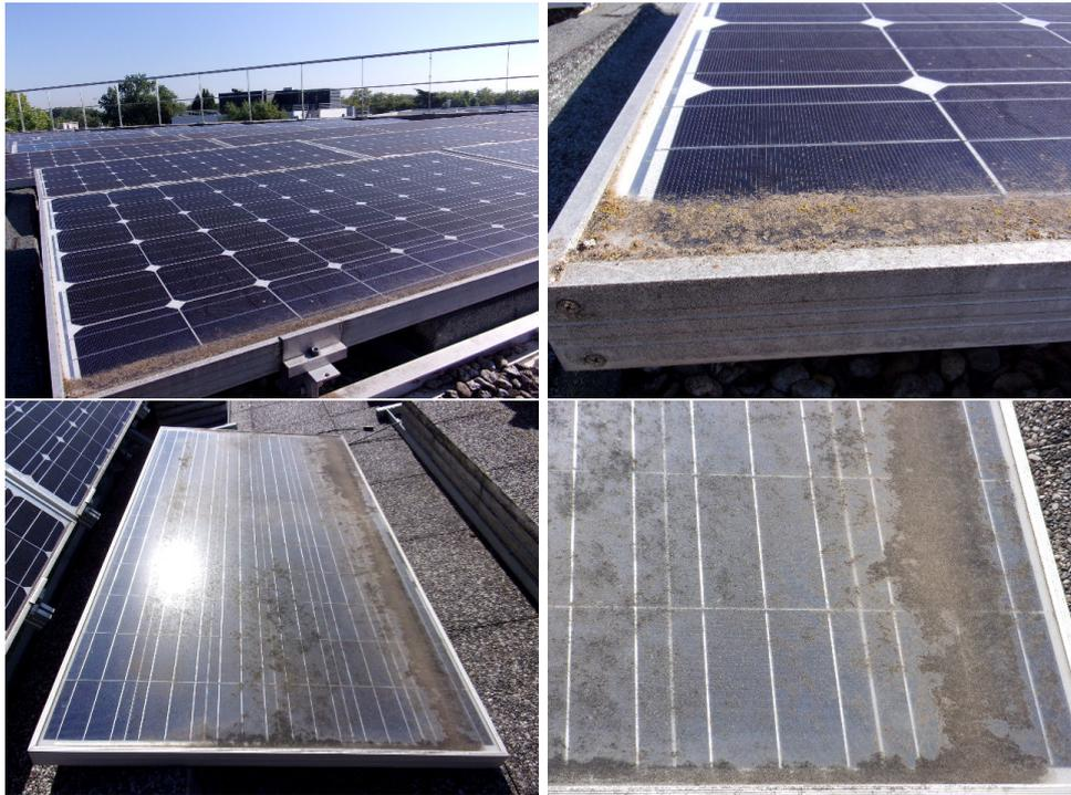
**Figure 1.16** Example of dust accumulation on a PV module
