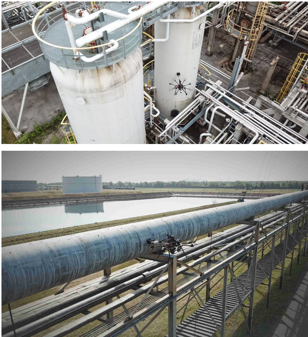
Figure 11.10 – The AeroX platform performing ultrasonic thickness measurements in a refinery located in Germany.
