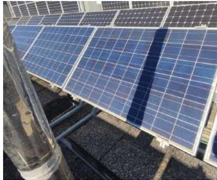
Figure 2.29: Example of Shading
