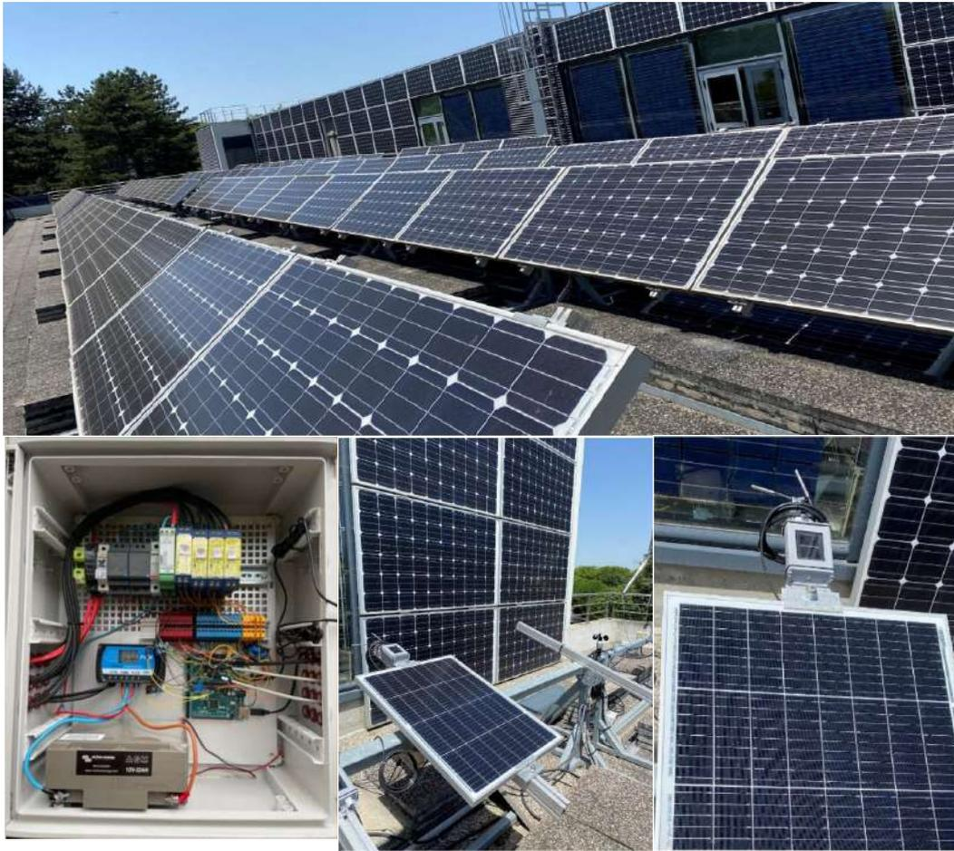
Figure 5.8: Installation of the third version of Solar Vitality in the LAAS-CNRS
